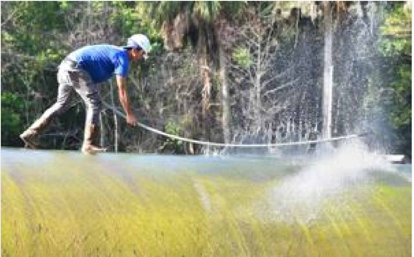
Water restoration projects underway on Homosassa River, King's Bay
