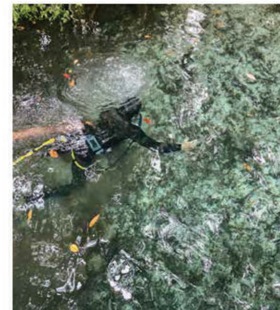
Sea & Shoreline diver dredges a river to remove muck from the bottom
